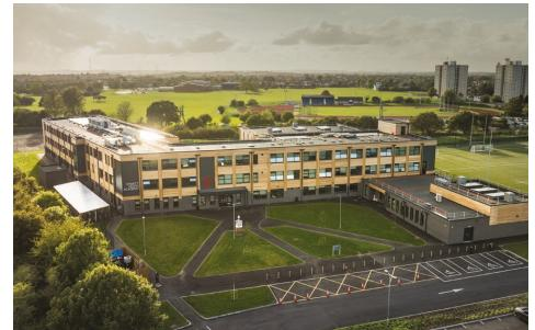
McAvoy provides complete turnkey solutions that adhere to the same regulations as traditional buildings but can be delivered up to 50% faster. Its modern, custom-built modules are typically more than 70% complete before leaving McAvoy's 70,000 square-foot purpose-built manufacturing facility in Lisburn, Northern Ireland. This facility has the capacity to design and manufacture up to 1,200 modules annually, making McAvoy one of the largest modular building providers in the UK.
